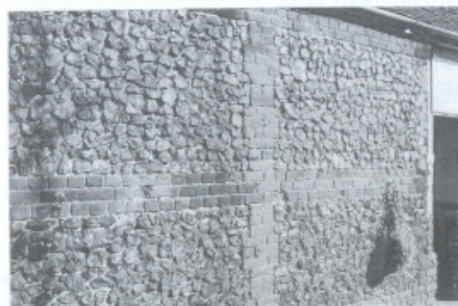
A wall of the stable block showing typical brick and knapped flint panels
